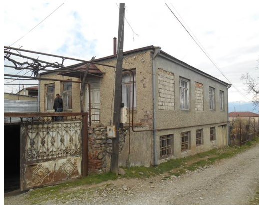
Private residential house in village Busheti
