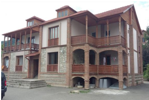
Two-story Residential Building (Antiochia Street #2)
