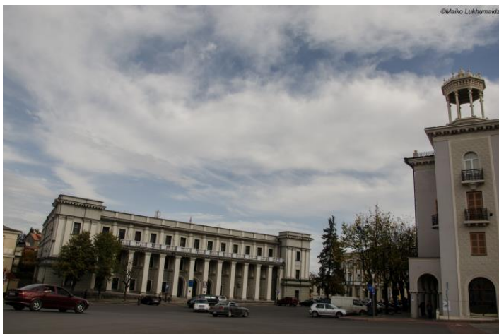
Figure 5. Administrative building of Telavi Municipality
