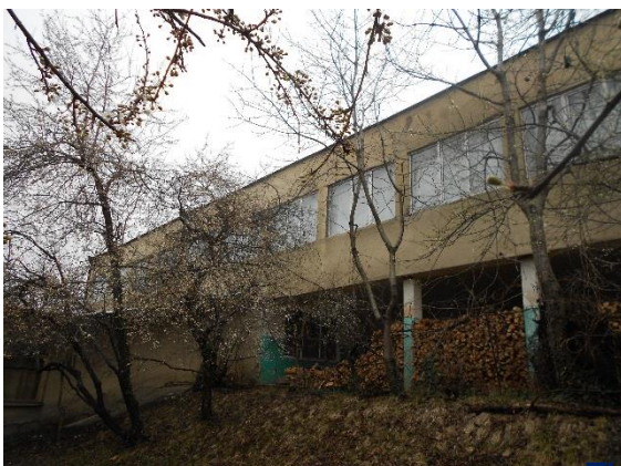
The Telavi #7 kindergarten; Address: 2A Alazani Ave.
